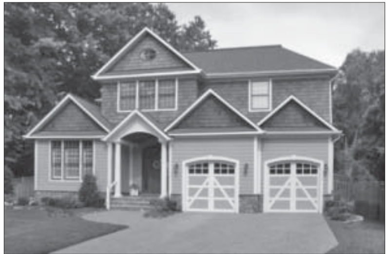
Result of a Design/Build project by Sagatov Associates.
